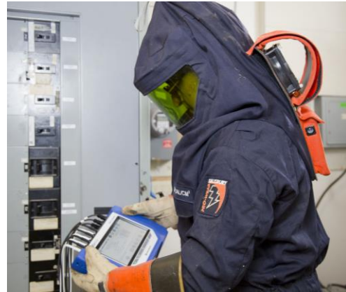
Figure 1. Portable power quality monitor being installed by an electrician wearing PPE clothing
